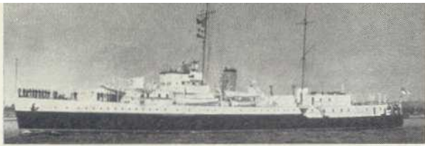
HMS Enchantress, completed as an Admiralty Yacht, was altered during her building. Designed to mount four 4.7 inch guns, she commissioned with three, but quickly lost No 3, which was sited just forward of her pole mainmast (Wright and Logan).
