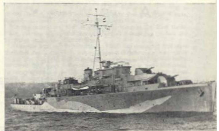
Cygnets features in the variants table. Here, the starboard quad pom-pom is clearly visible abaft the funnel. Notice her tripod foremast and 'crowsnest'. Left: Most famous of the class was Amethyst , here seen returning shell-scarred from the Yangtze action in 1949. Note the 'plugged' shell holes near the waterline.
