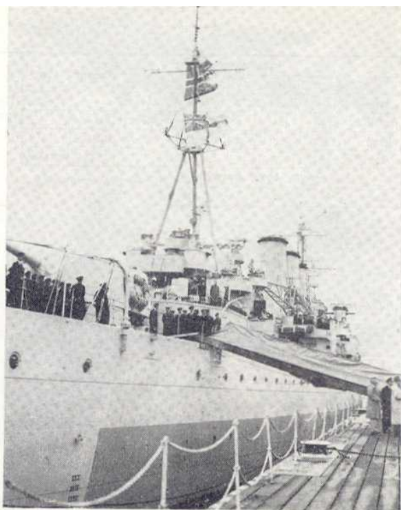
HMS Norfolk in 1945. A veteran of the Bismark and the Scharnhorst actions, she was chosen to convey King Haakon back to Norway after his war-time exile in UK. Many of the equipments discussed in this series can be seen in the photograph. 'X' turret has been replaced by a pair of 'quad' pom-poms, with sided directors abaft the tripod mainmast. Superimposed above them is 'Y' turret's Barrage Director. Forward of the mast is the 8 inch Director Tower and a Height Finder Radar in the old HACS Director position. There is a pom-pom director for the starboard 8-barrel weapon just outboard of the 8 inch DT and the starboard director of the revised HACS layout is visible abreast the bridge superstructure.
