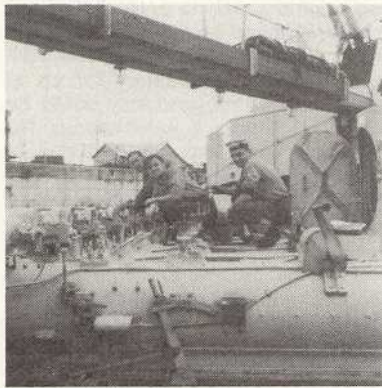
Maintenance work in progress on a set of 'Pentad' torpedo tubes. The door of the cupola is open and a catwalk runs over the tube mounting linking the gundecks. The 'signal box' style lever operated the tube training locking bolt, and the hand-crank was the alternative method of training the tubes outboard to the firing position (Anthony Peters).
